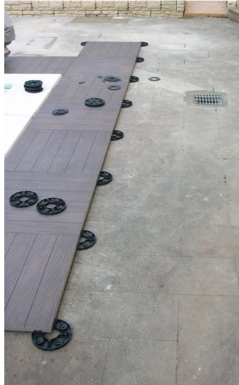
fixed height support pads (1/2" to 1" high) The pedestals can be taken apart.
