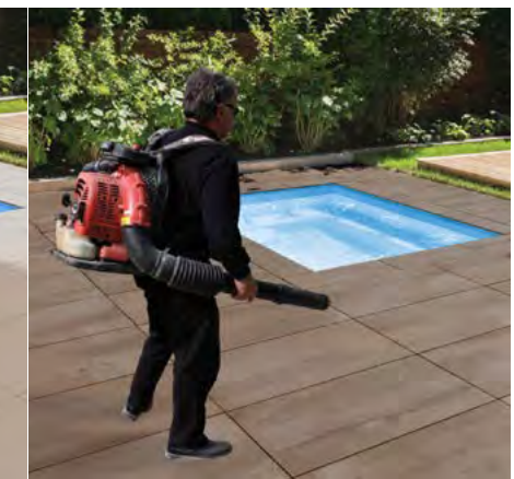
5 Sweeping, compacting and blowing of the tile sand.
