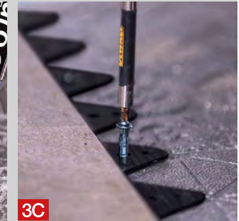
3C Installation of Euro Tile Edge and Euro Base Screws
