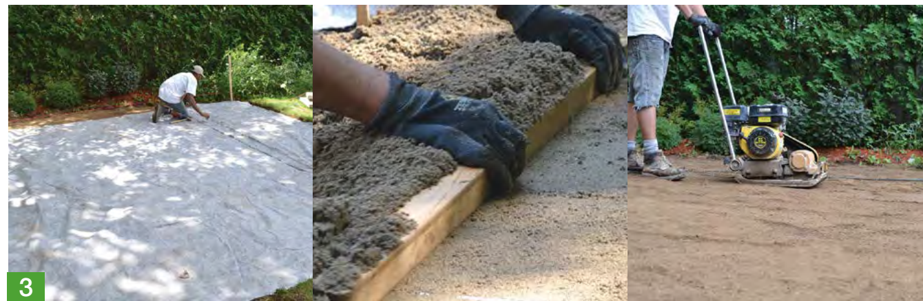
3 Addition of geo-fabric, levelling and compacted bedding sand
