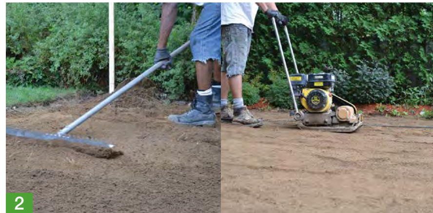
2 Levelling and compacting of the base
