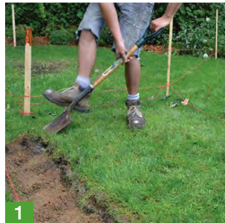
1 Excavation of the new area.
